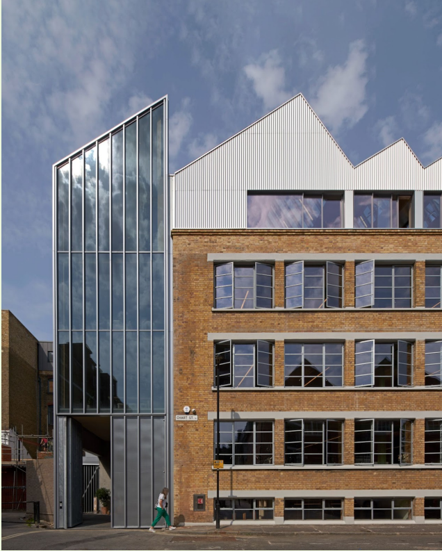
16 Chart Street, Hackney Design Awards Winner 2022 (new build elements in sustainable structural timber)
